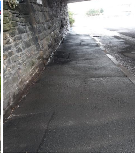
Amberley Rd Rail bridge clean-up
