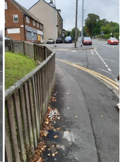
Swinnow Road Asbestos
